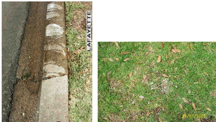
Figure A-100. Left: Exfiltration onto the Pavement (Section #7). Right: Surface Exfiltration onto the Grass (Section #9).
